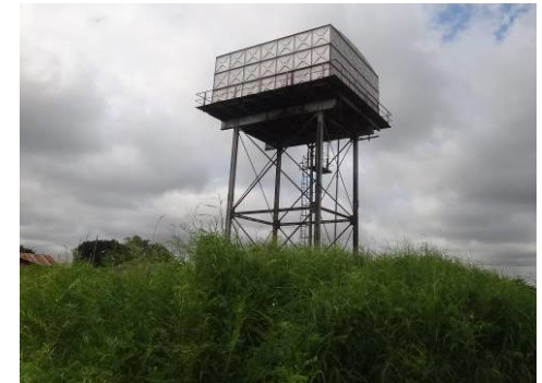
Elevated Water Tank
