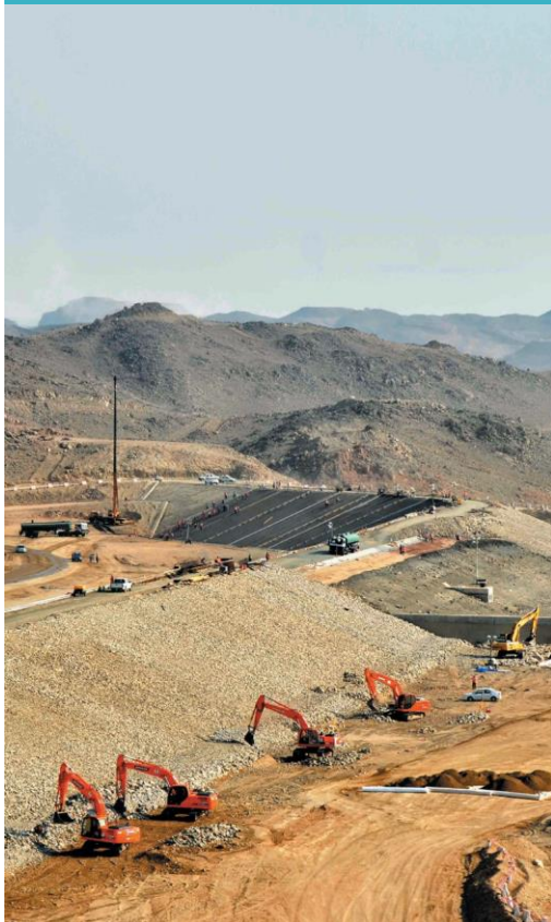
Jeddah Storm Water Project / KSA
