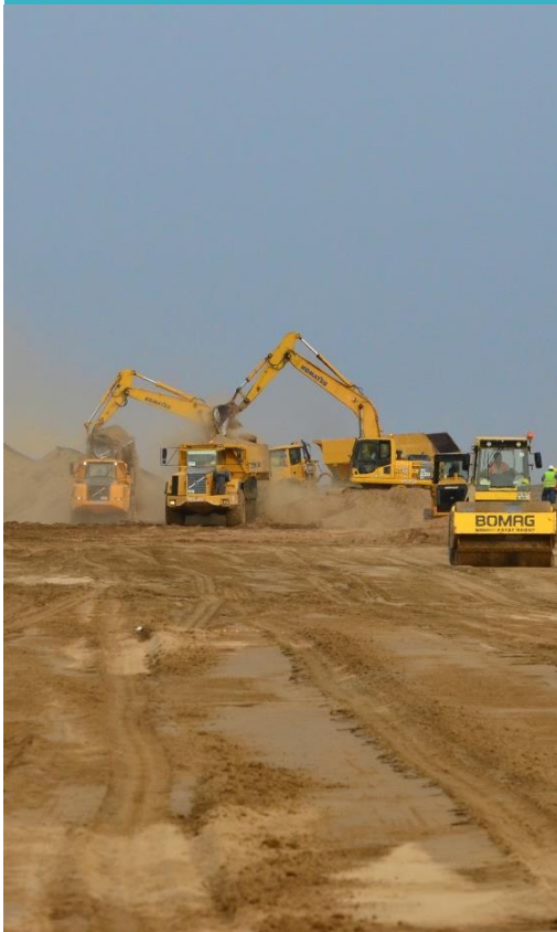
Jazan Economic City Site Development Project / KSA
