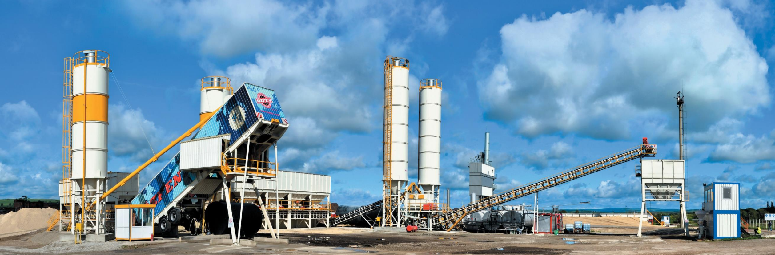
Chisinau Soroca Road Project Production Facilities / Moldova
